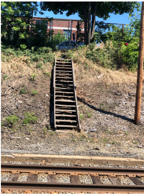
8. Steps to a locked Washington St gate
