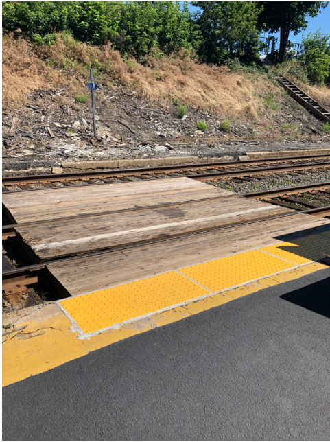
7. Walkway to access the north side track
