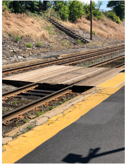
9. Walkway and steps in one photo
