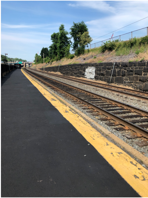
11. View west towards the end of the old north side platform
