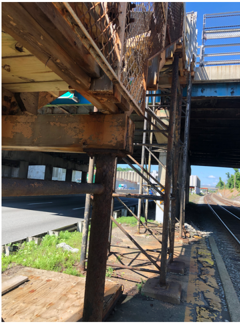
4. Underneath the Walnut St stairs
