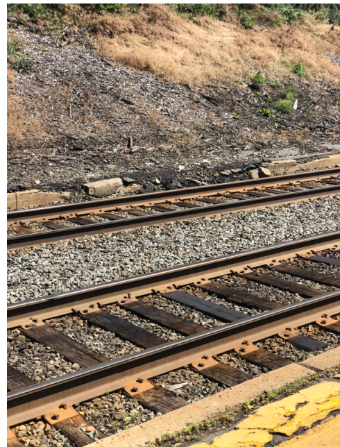
6. Section of the north side platform in disrepair
