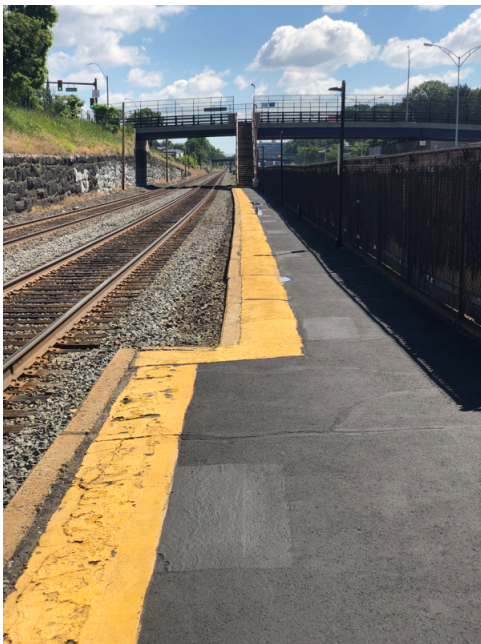
13. Closer view east towards Harvard St
