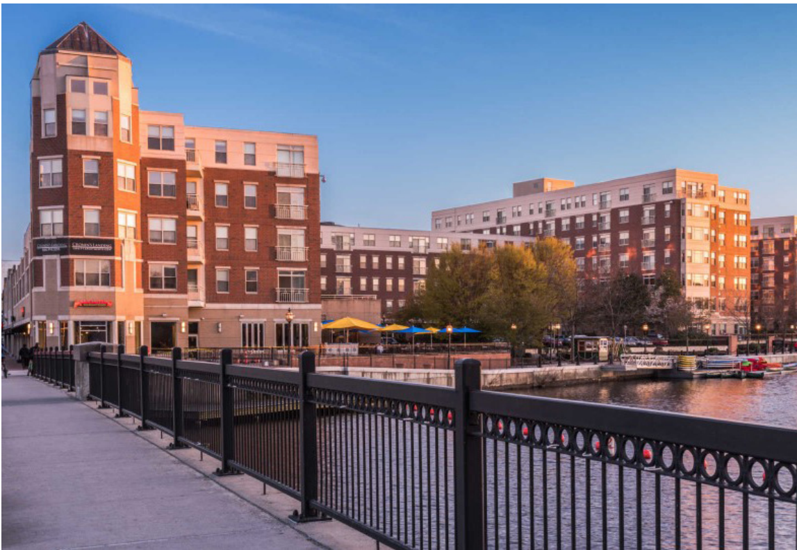
Cronin's Landing Apartments overlooking the Charles River in Waltham, MA near Waltham Commuter Rail Station. This project is a good example of a mixed-use building located a short walking distance from a Commuter Rail line.
