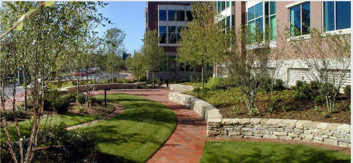
Landscaping in front of Riverside Center at 275 Grove Street. Source: CRJA-IBI Group
