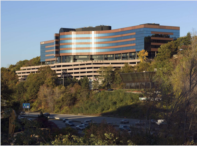
View of CityPoint from I-95/Rte. 128 that shows the structured parking incorporated into the topography.
