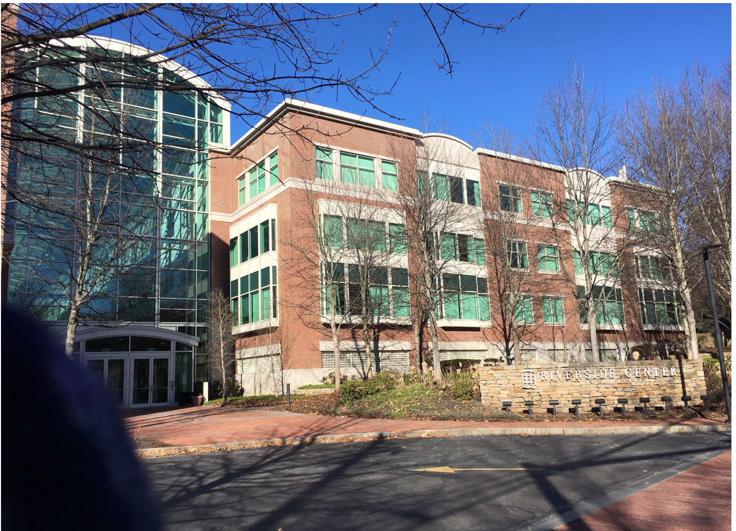
Riverside Center, a commercial office space that contributes to Newton's commercial tax base, is situated directly north of the Riverside site.
