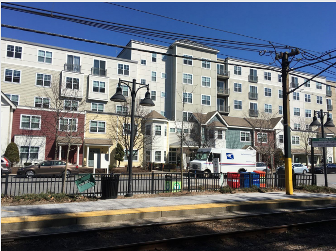
Apartments at Woodland Station along the D Branch of the MBTA Green Line.
